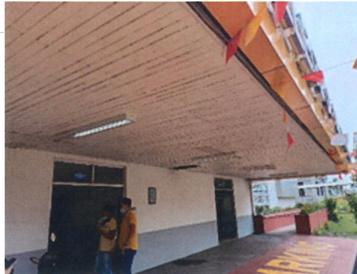
EXISTING CEILING CONDITION
